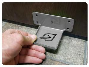
Position Footplate at the lower corner, on "pull" side of door and mark hole locations.
