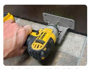
Starting with the center hole, drive the (three) #10 Mounting Screws into door.
