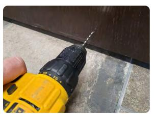
Using a 1/8" drill bit, drill (three) starter holes for the #10 Mounting Screws.
